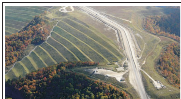
King Coal Highway, West Virginia (Special Negotiated Agreement). Some construction work for this 90-mile, four-lane highway is being done by local mining companies as they extract coal nearby. (Photo: FHWA)
