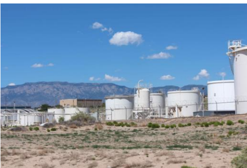
South Valley Oil Facility
