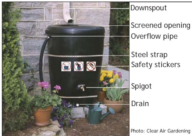
Figure 13. Components of a passive rainwater harvesting system
