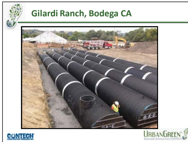
Figure 24. California ranch cistern system
