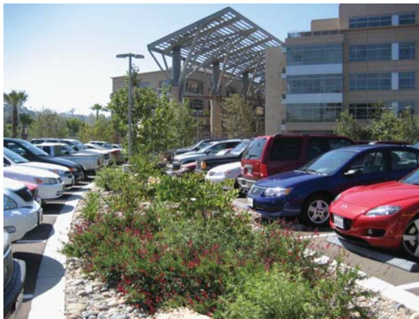
Figure 6. Bio-retention of parking lot runoff in San Diego
