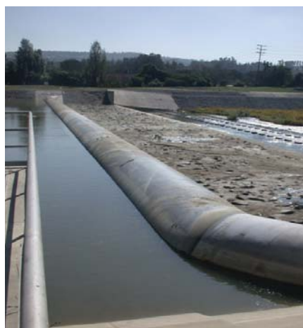
Figure 4. Inflatable dam diverting water from the Santa Ana River
