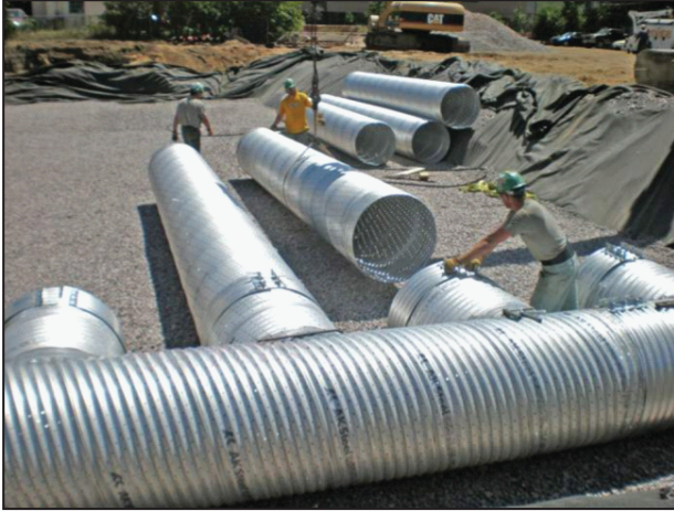
Figure 19. Impermeable pond liner in the background and perforated metal pipe that will be filled with gravel and wrapped over the top, similar to the chamber system
