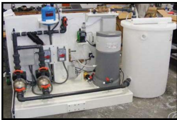
Figure 15. Traditional active mechanical rainwater harvesting components
