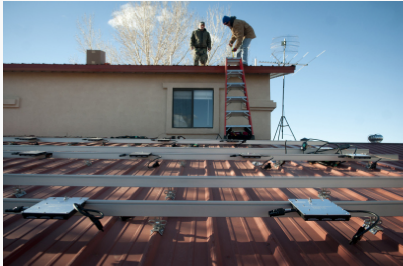
Patrick Griebel of Affordable Solar says PNM's proposed fee structure could kill the rooftop solar industry.
